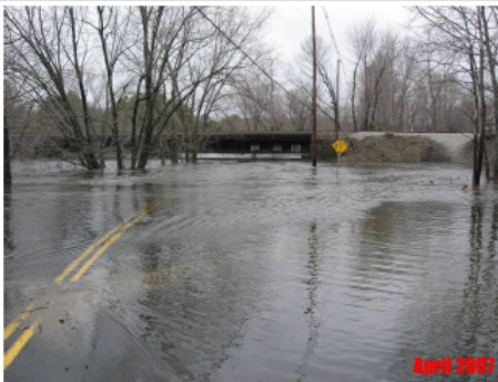
MACPHERSON ROAD AT RAILROAD BRIDGE VIEW NORTH
